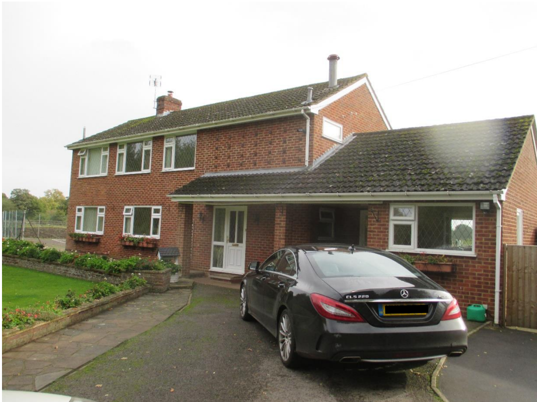
Existing dwelling and garden
